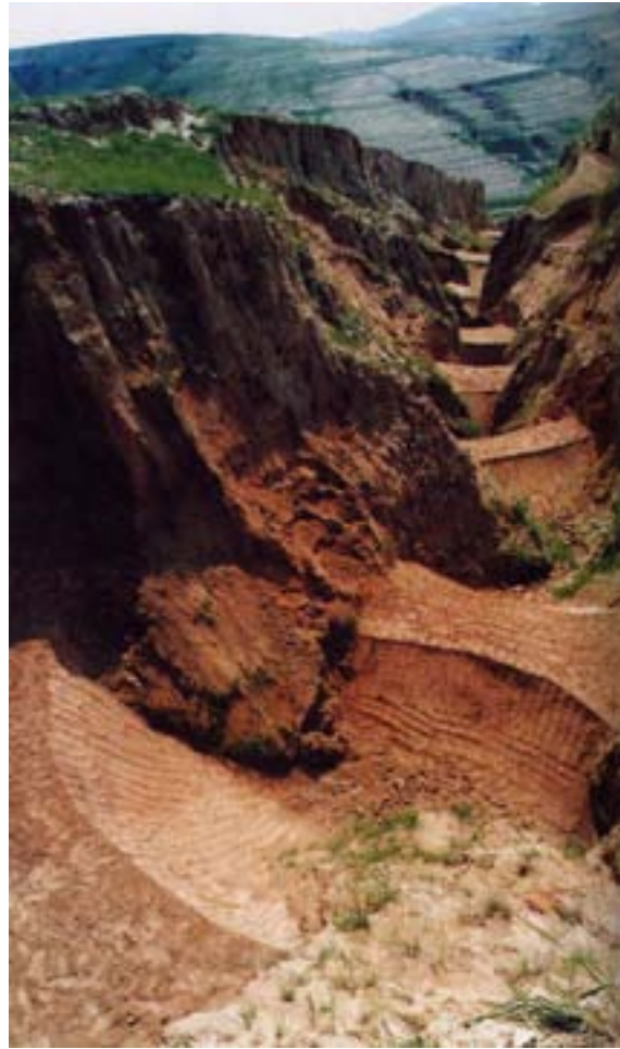
Photo 4 Earth check dam in Shanxi Province
