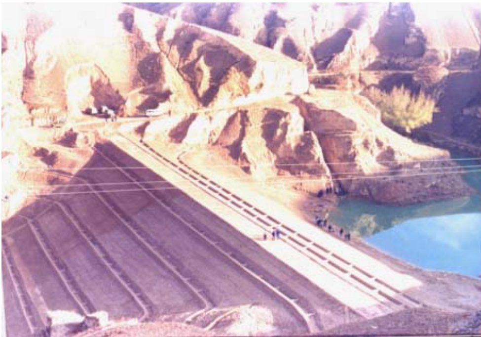
Photo 3 Warming dam just completed on Gully, Shaanxi province
