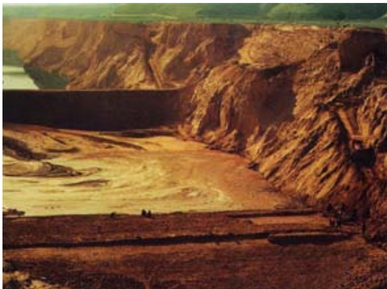
Photo 5 Hydraulic fill dam in Shanxi Province
